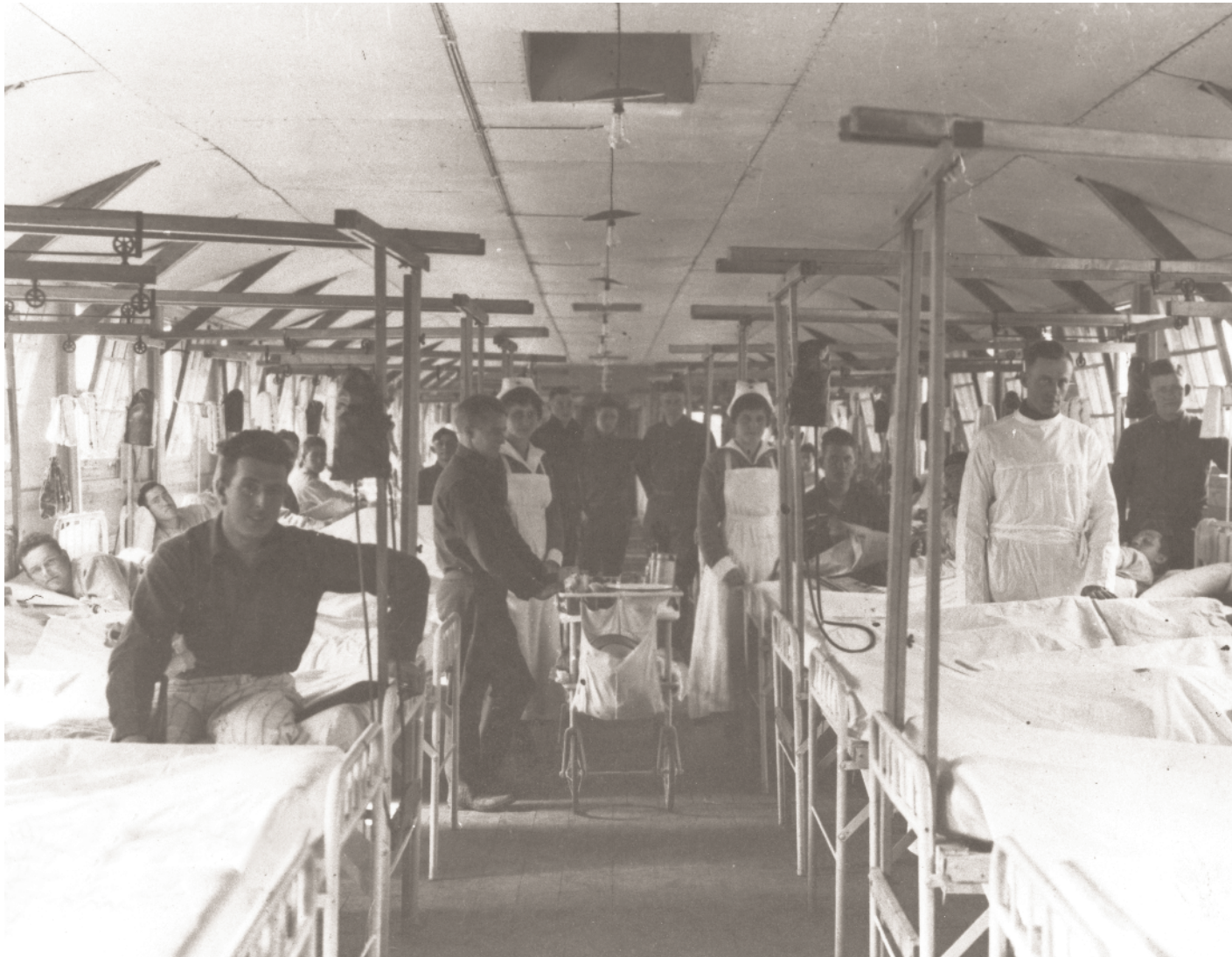
Ward of Evacuation Hospital No. 20 showing Balkan frames.
